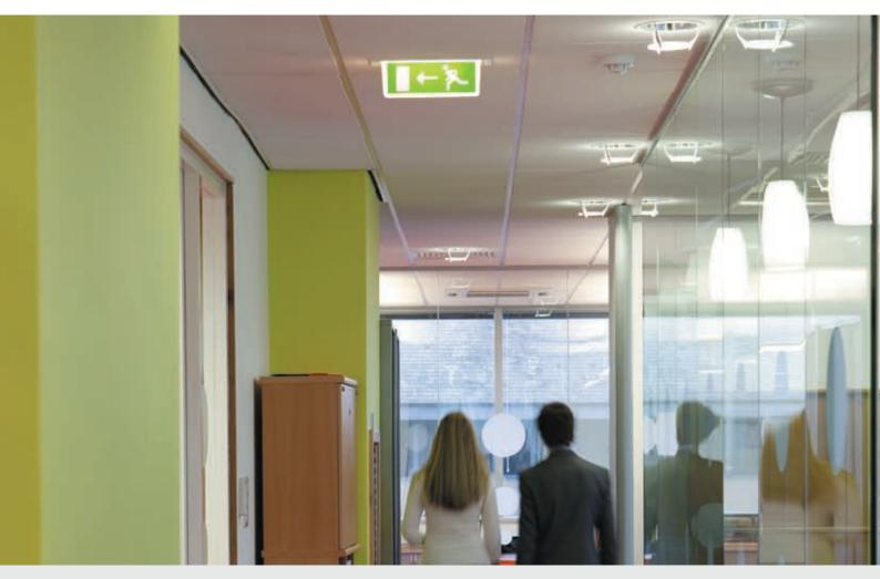
**Solution**Voyager LED Route luminaires use special optics to comply with regulations and ensure clear visibility of the escape route. The optic is mounted axially in line with the escape route for maximum performance.
